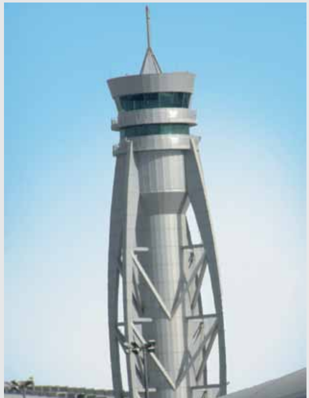
Airport Control Tower, Dubai
