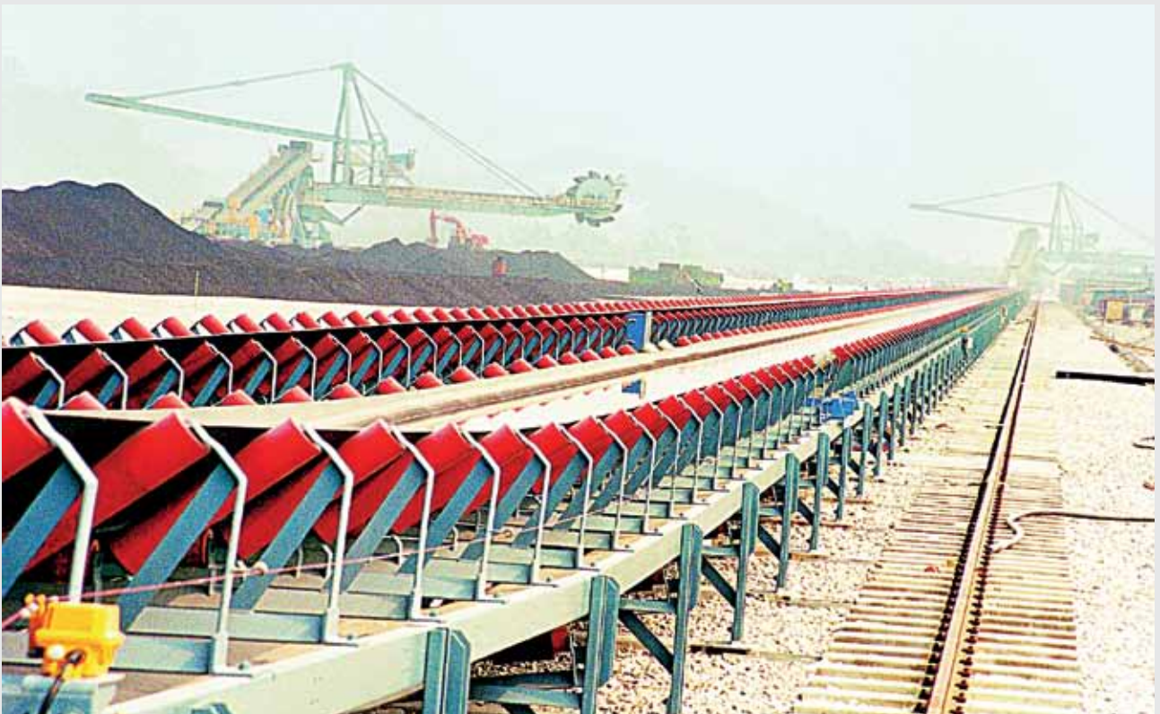
3 X 700 MW Manjung Power Plant, Malaysia - Stockyard
