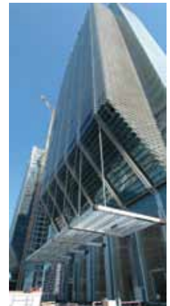
Sowwah Square – Tower Canopies, Dubai
