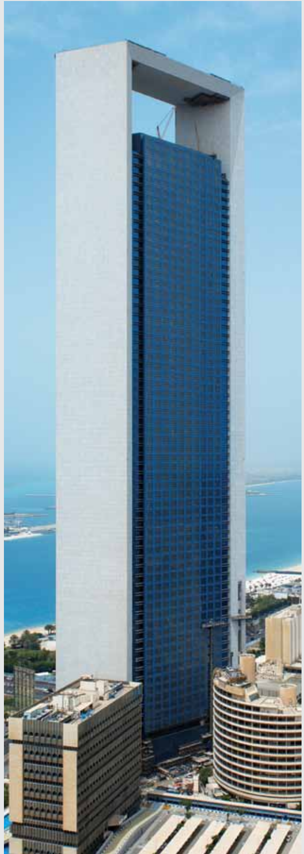
ADNOC Headquarters, Abu Dhabi
