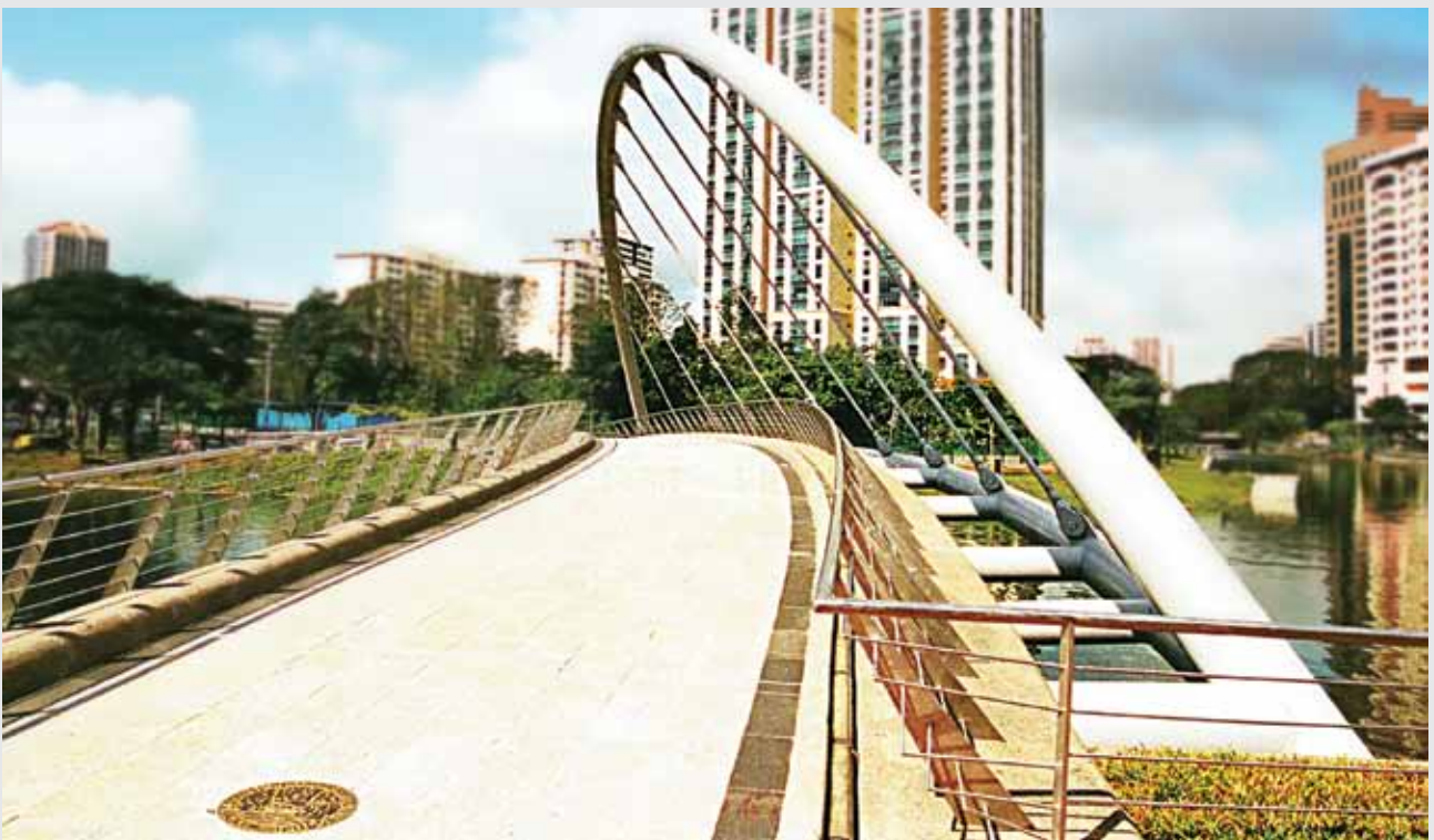
King George's Foot Bridge, Singapore
