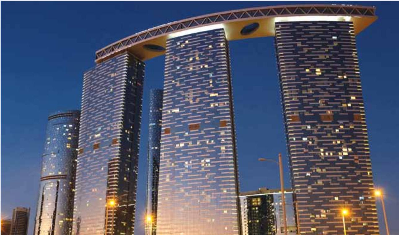
Gate District Towers, Abu Dhabi
