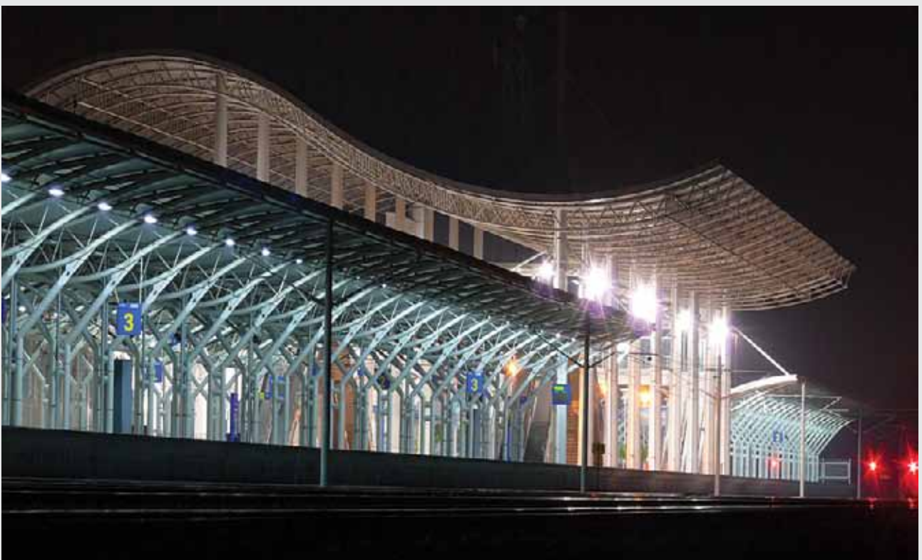
Rawang - Ipoh Double Track, Malaysia
