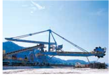
Stacker Reclaimer, Malaysia
