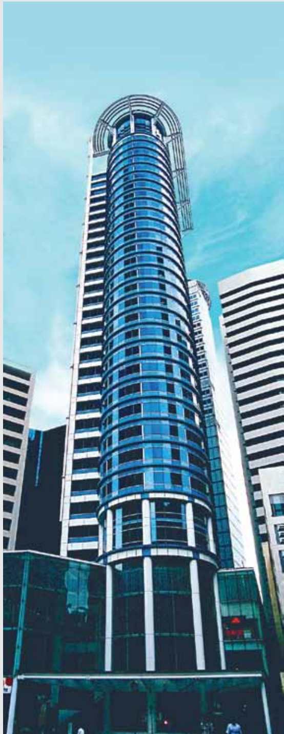
Caltex Tower, Singapore
