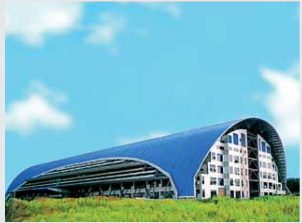
TNRD Bangi Project, Malaysia
