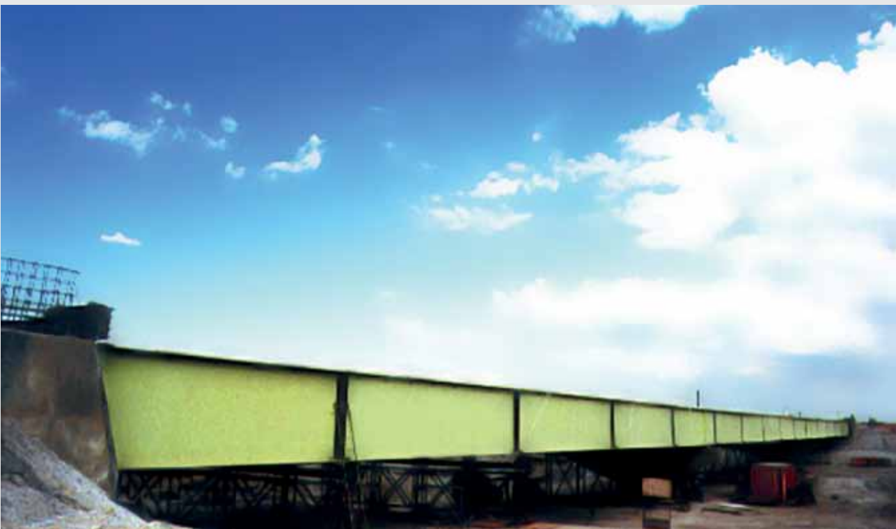
Mabalacat Bridge, Philippines
