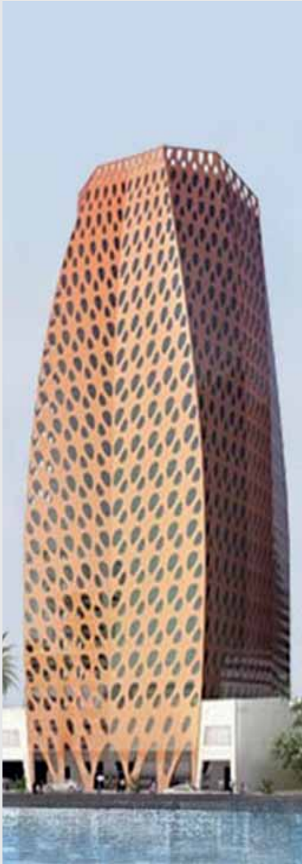
Al Nasser Headquarters, Abu Dhabi
