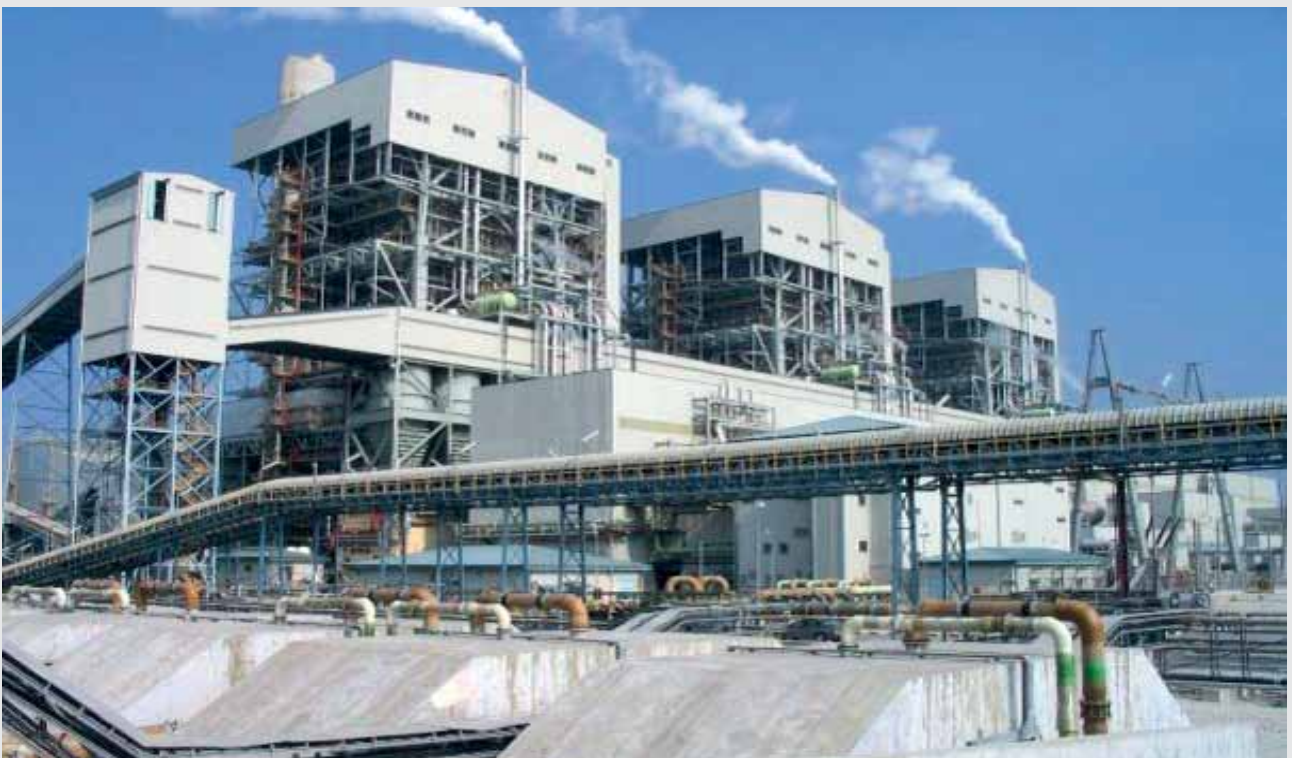
3 X 700 MW Manjung Power Plant, Malaysia
