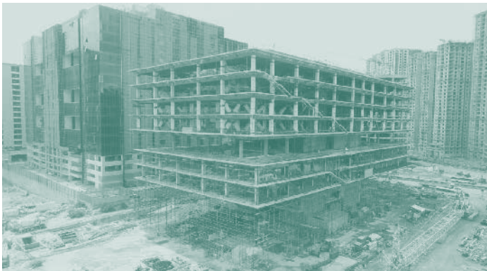
T Hub Phase II, India.
