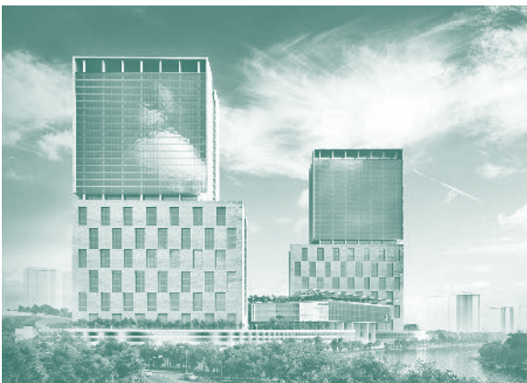
Sands Infra IT Building, India.
