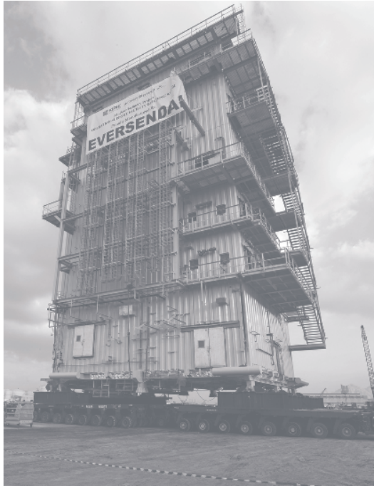
KIPIC Building, Kuwait
