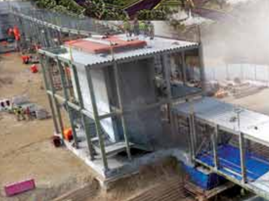
Al Jalila Hospital Link Bridge
