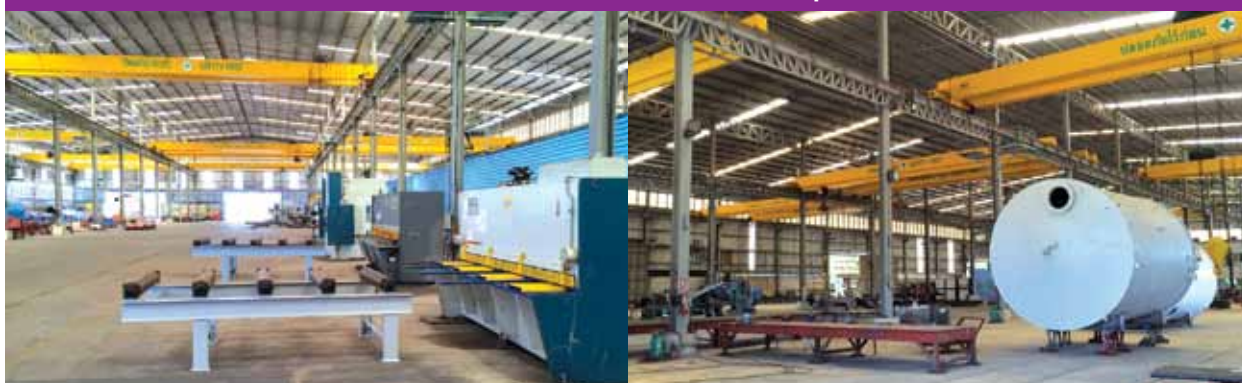
Eversendai Thailand's fabrication plant
