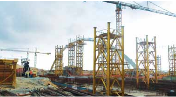
• King Abdulaziz International Airport – Railway Station, Saudi Arabia
