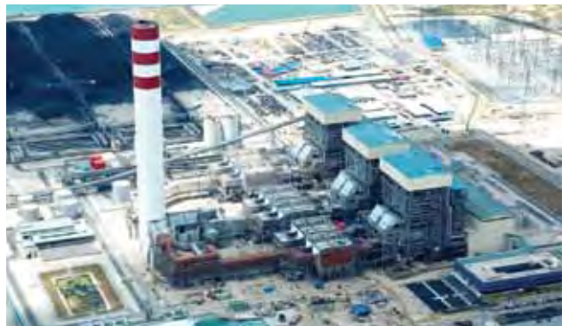
Tanjung Bin Coal Fired Power Plant, Malaysia
