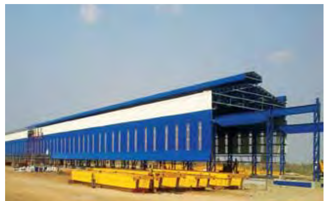
Fabrication Yard, India
