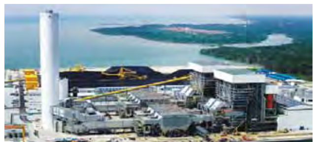
Jimah Coal Fired Power Plant, Malaysia
