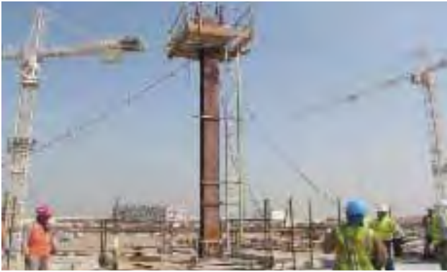
August 28 Start of Erection – Yas Mall Abu Dhabi, UAE
