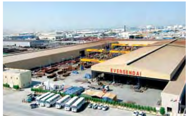
Fabrication Yard, Hamriyah
