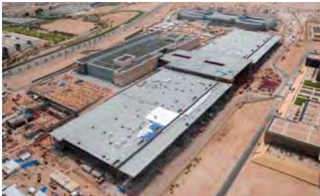
Qatar National Convention Centre Extension
