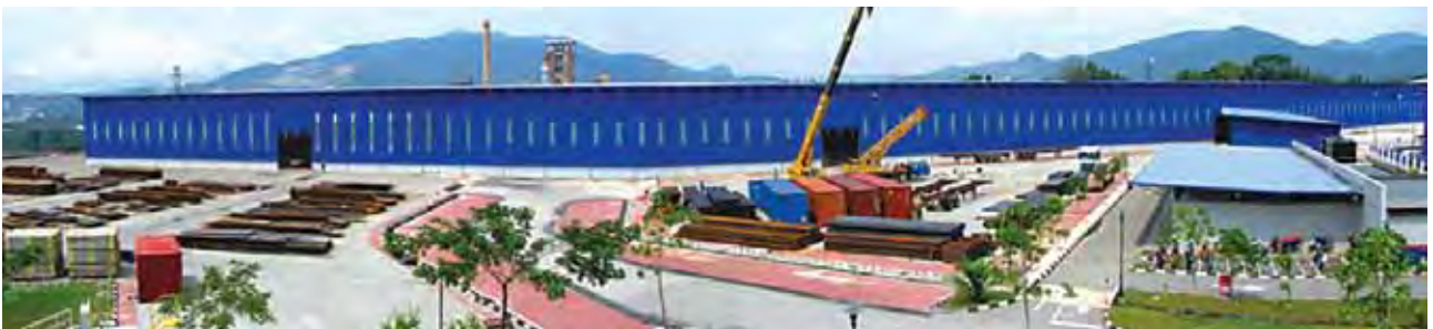
Fabrication factory in Rawang, Malaysia
