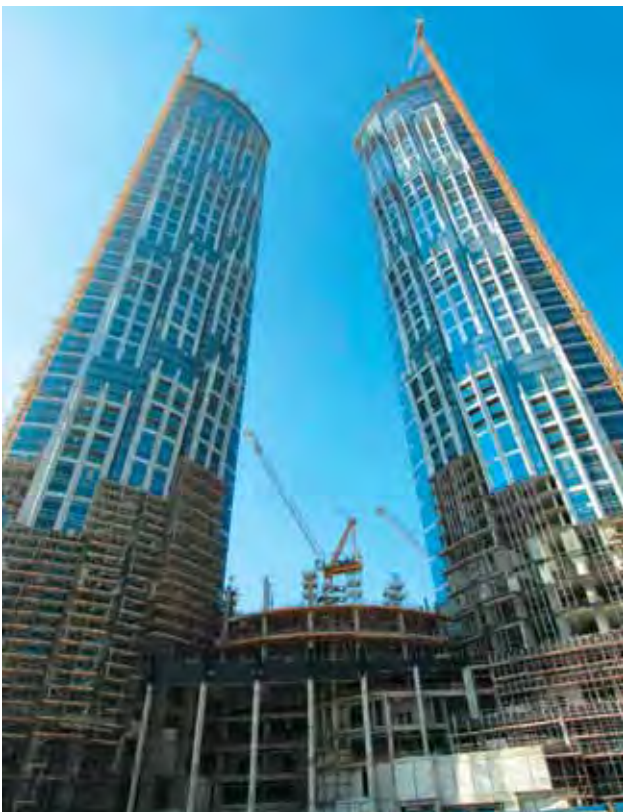
Emirates Park Tower Hotel
