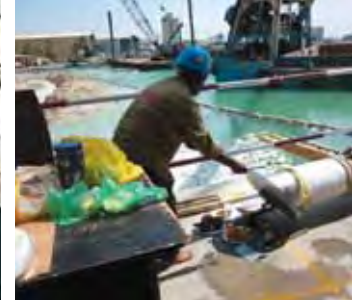
13 October 2011 Start of Erection Dubai, UAE
