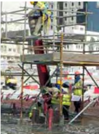
National Museum of Qatar Start of Erection Qatar
