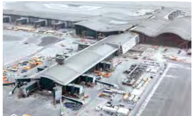
New Doha International Airport (NDIA)
